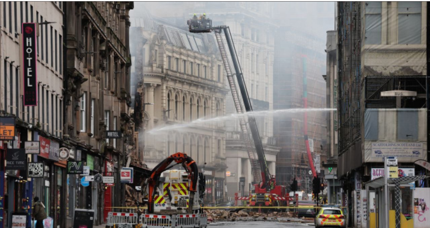
Glasgow: Due to a fire that destroyed a nearby building on Sunday, Glasgow Central station's high level will be closed for the remainder of the week. Due to the fragility of the mid-Victorian block on the intersection of Union Street and Gordon Street, much of
